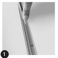
Drill holes for screws (2 per 500mm/20") and rear cable entry (10mm/0.39" min.) and coat raceway with corrosion inhibitor if required.
