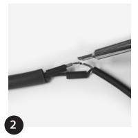
Make power connection to suit IP requirements of installation location. Adhesive lined heat shrink recommended for compact joints in raceway.
